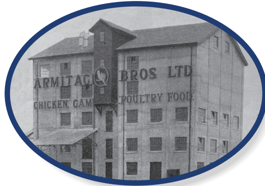
1924 - New mill opened at Colwick
